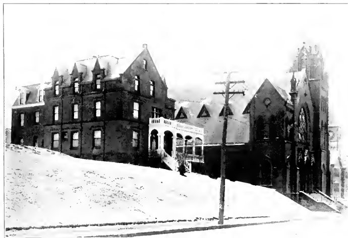
ST. FRANCIS XAVIER'S CHURCH AND RECTORY, WATERBURY
